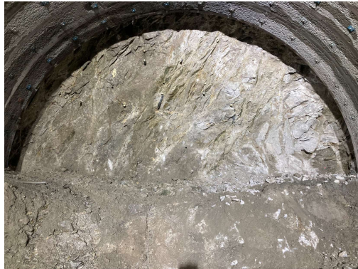
斜坑_切羽状況_0k825m
